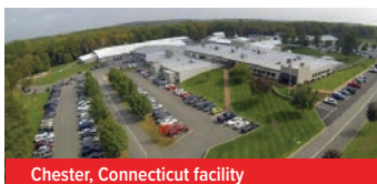
Chester, Connecticut facility
